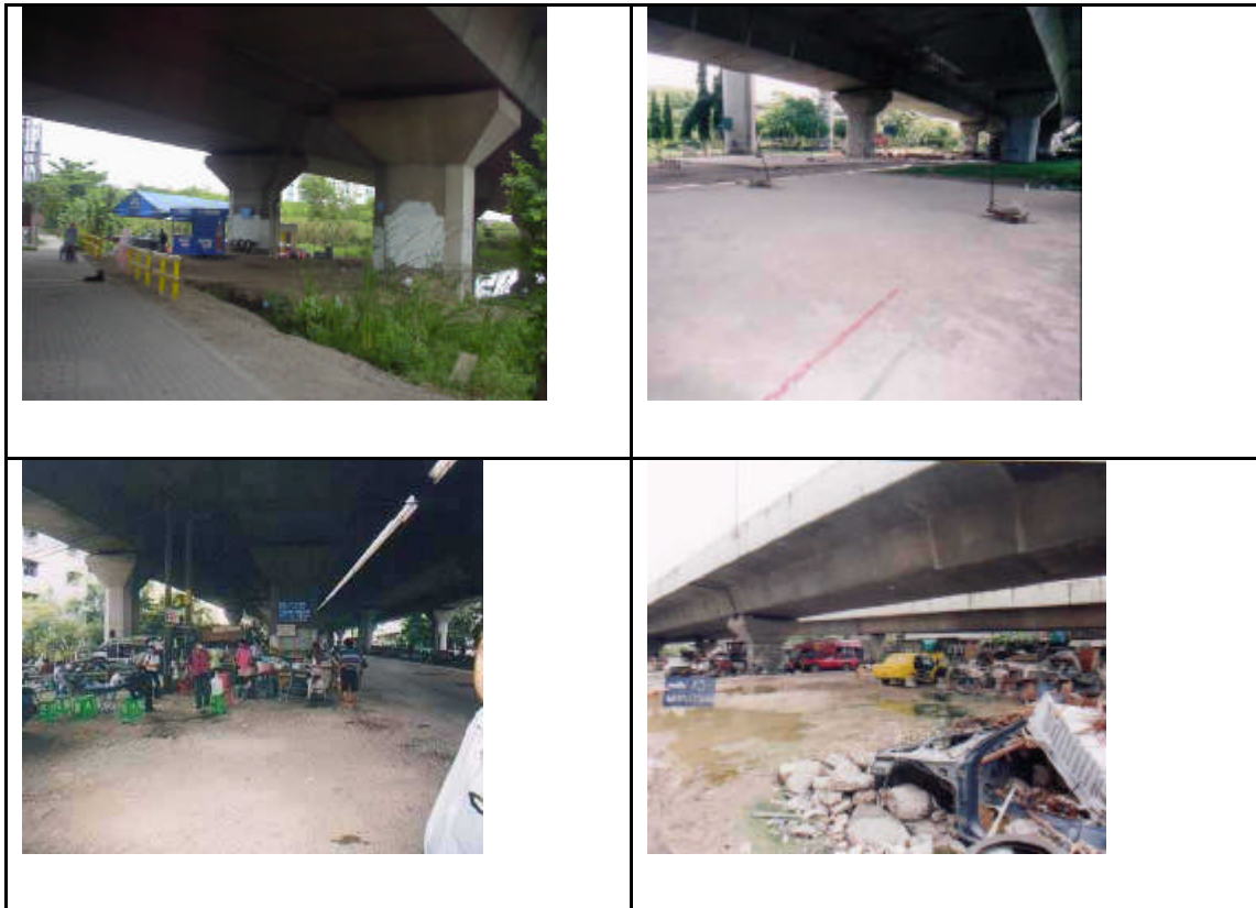
Figure 17: under-utilized land under elevated expressway
