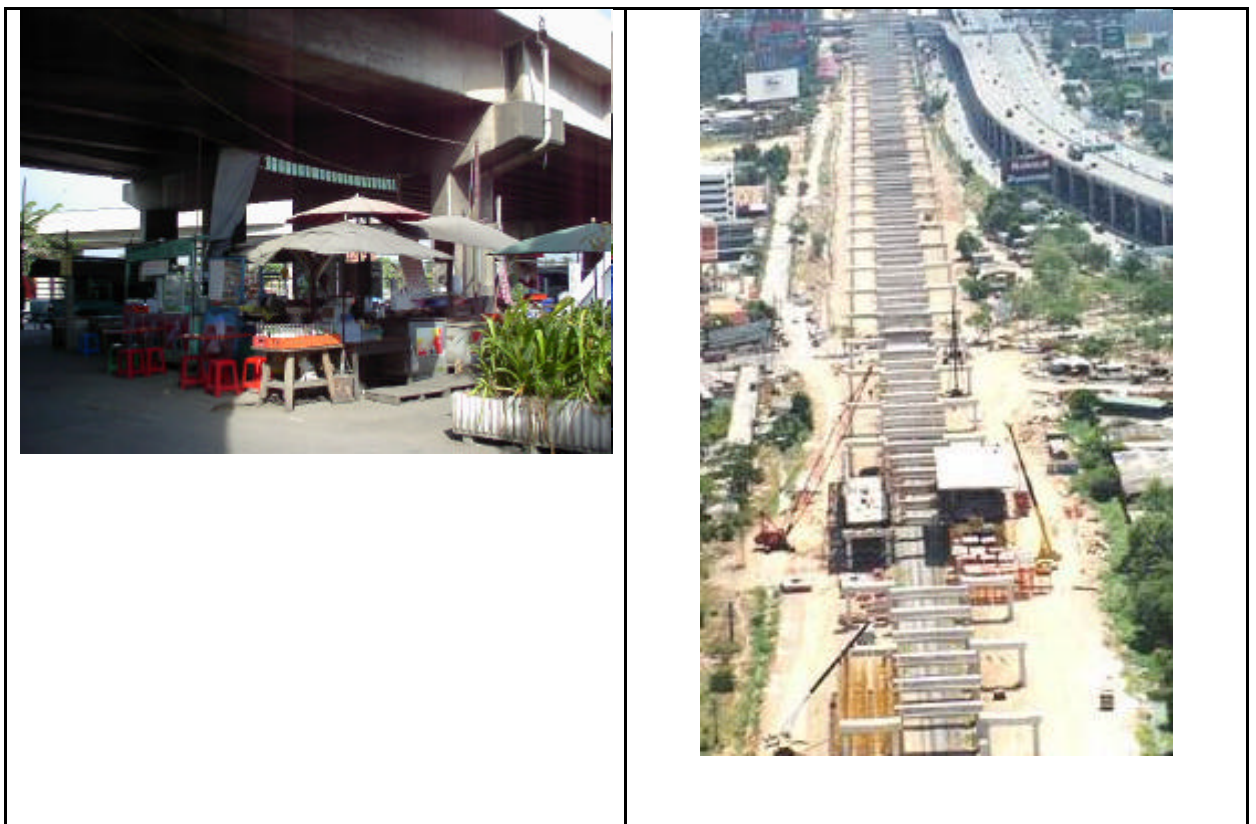
Figure 18: under-utilized land under the elevated road/bridge and under and along the Hopewell / rail line
